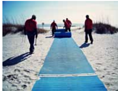
Un-rolling prior to installation
