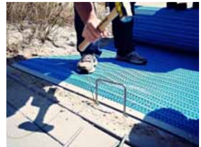
Pinning down the ends
