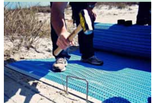
FIG. 2 - ANCHOR THE PATHMAT END WITH U-PINS
