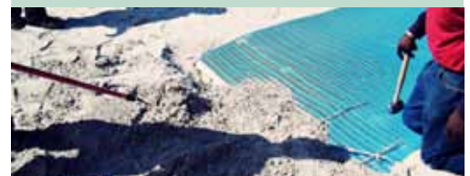
FIG. 3 - COVER ENDS WITH SAND TO PREVENT TRIPPING
